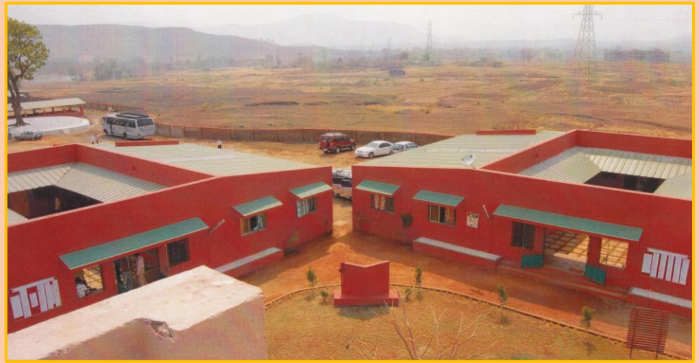
AERIAL VIEW OF THE PROJECT
